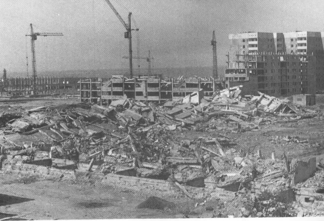
Damage to apartment buildings in Leninakan (present-day Gyumri) caused by 1988 earthquake Courtesy John Filson
